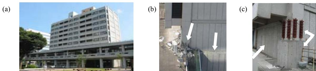
Photo 1. (a) Objective building, (b) crushed column, and (c) emergency rehabilitation
