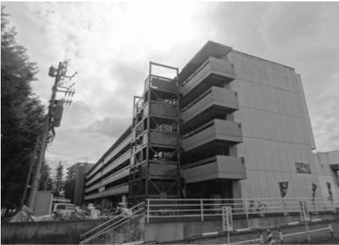
Photo 1. Panoramic view of building A
