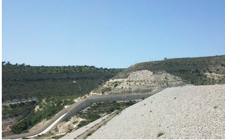
Figure 3: The downstream shell and right abutment.
