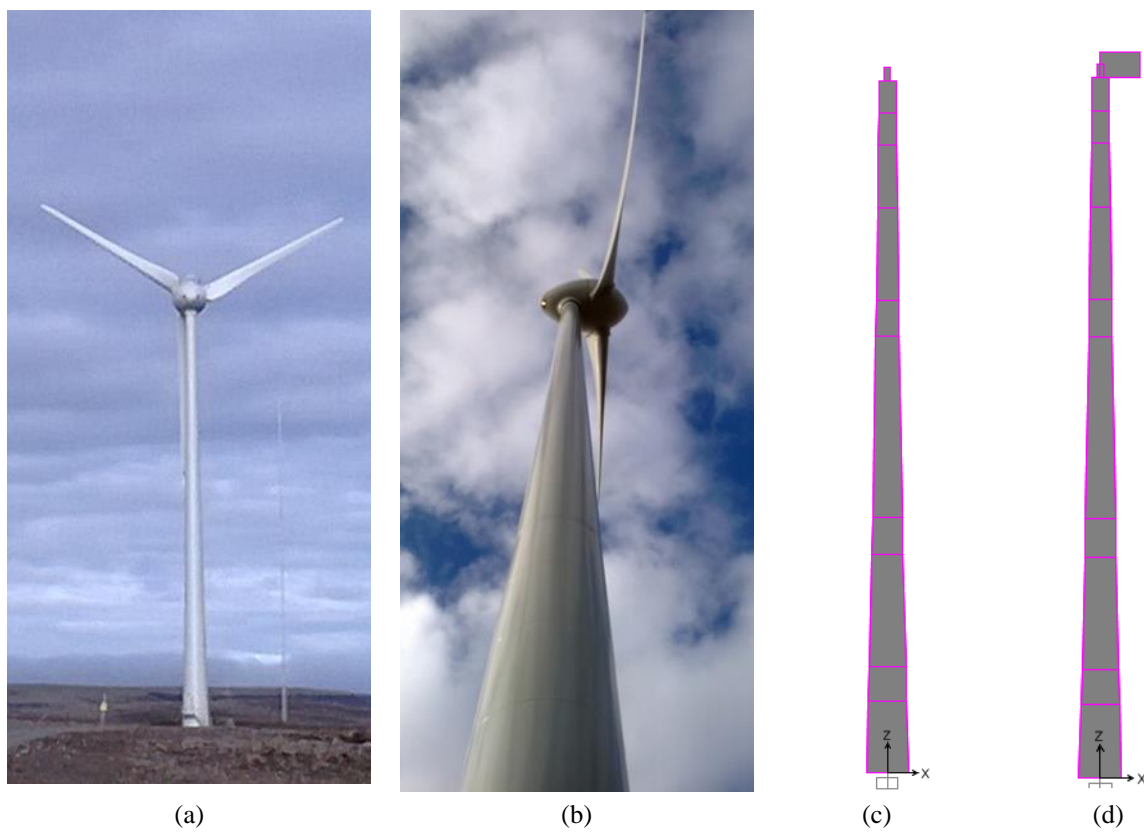
Figure 1. The study wind turbine: (a) the wind turbine in the natural surroundings; (b) view of the nacelle, (c) FE model without excentricity; (d) FE model with excentricity.
