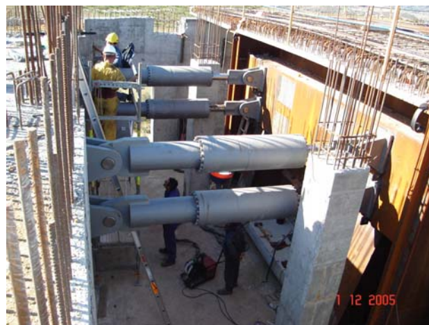
Figure 2: Hydraulic Viscous Dampers, an example of velocity Dependent Devices
