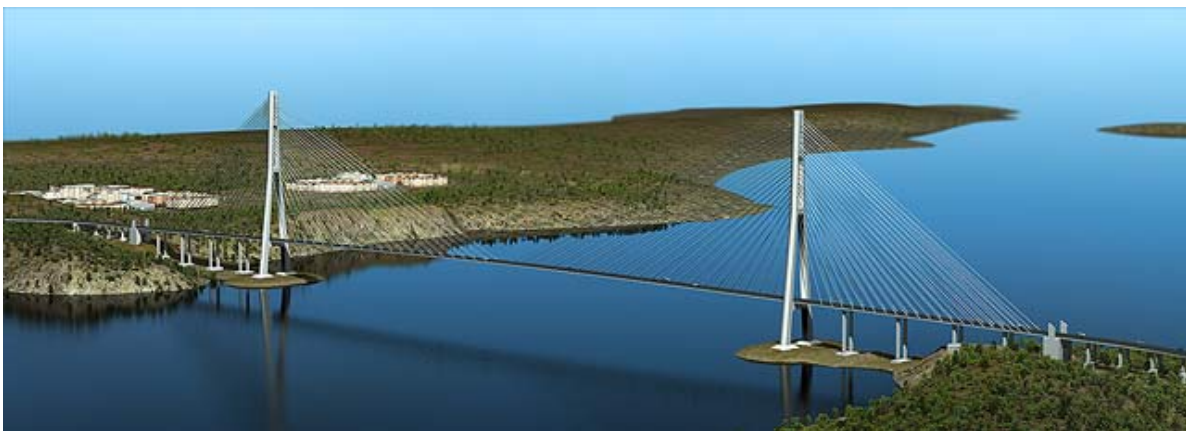
Figure 8: Cable-stayed Russkij Bridge – Vladivostok - Russia
