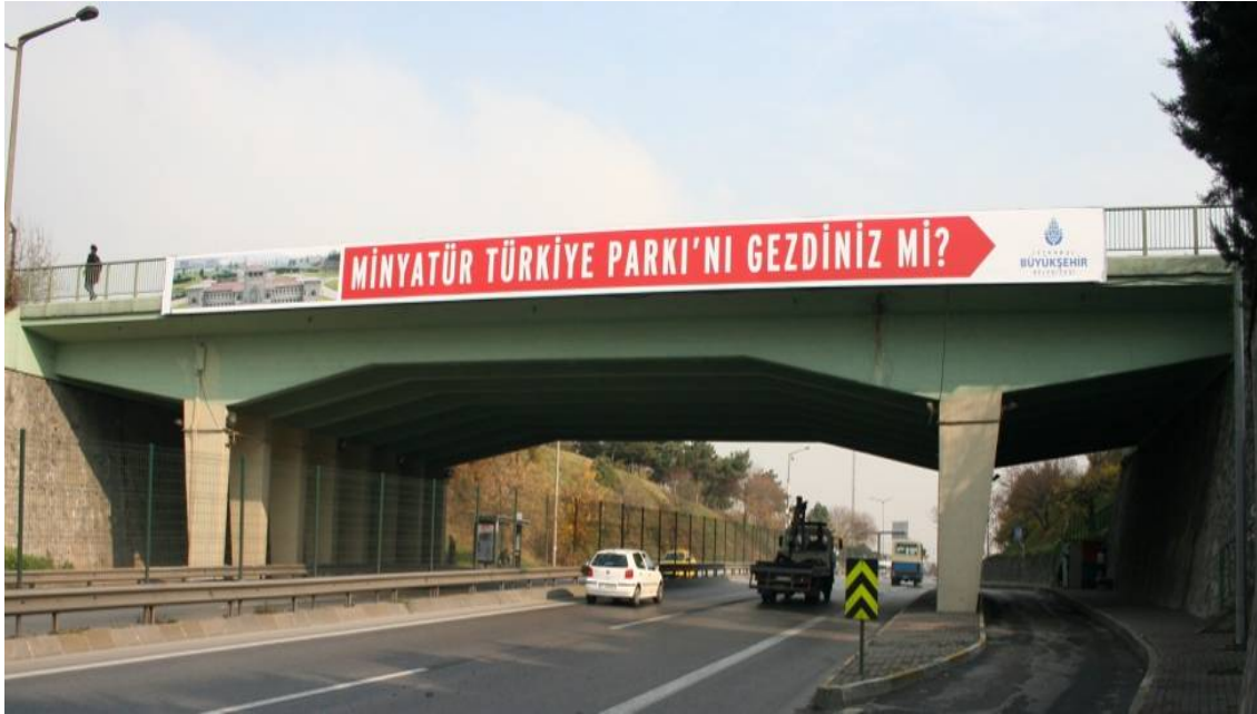
Figure 2.6. General view of Üsküdar-Haydarpaşa Overpass Bridge
