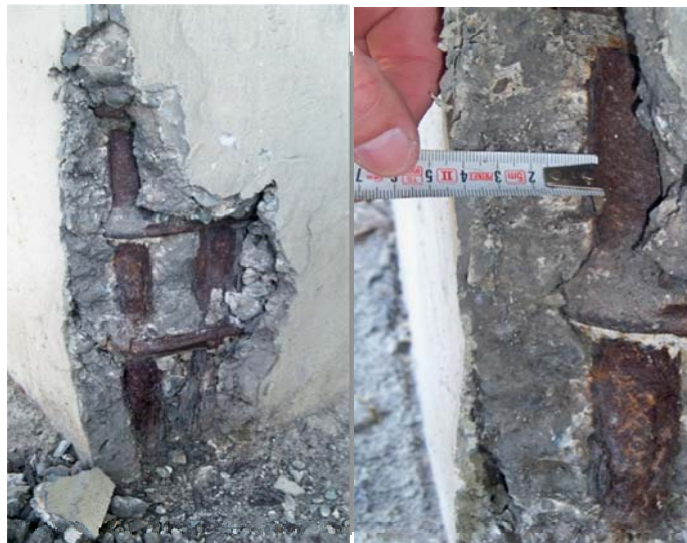
Figure 2.8. Measurement of existing steel rebar diameters at piers. (Üsküdar-Haydarpaşa Overpass Bridge)
