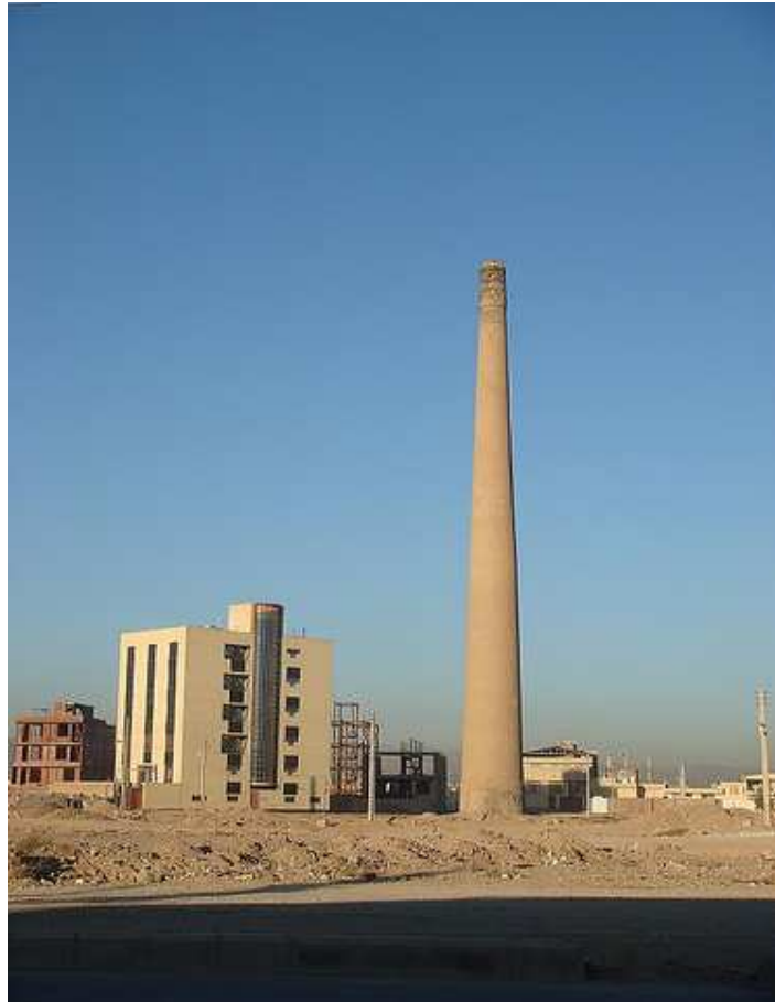
Figure 2. Industrial masonry chimney in Semnan (Iran)
