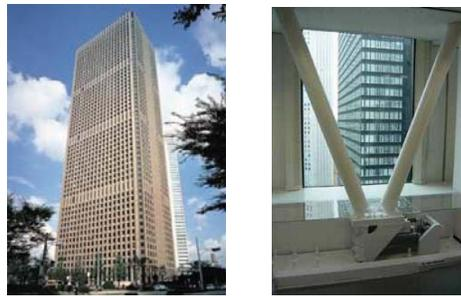
Figure 6 (Left) Picture of Shinjuku Center Building , and (right) dampers installed in 2009 [27].
