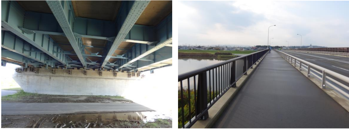
Figure 2. Details of girders and view of bridge deck
