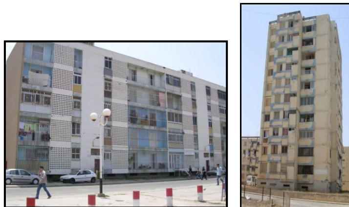
Figure 3. Building of three blocks in Cité 1200 logements (left), Building of 10 stories in Cité 800 logements (right)
