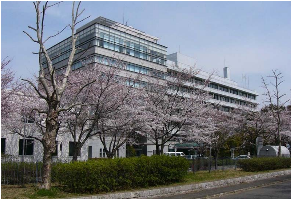
Figure 1. BRI main building (right) and annex building (left)
