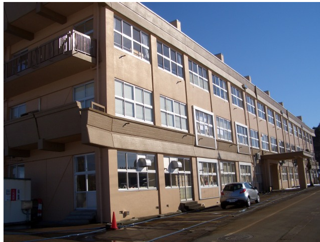
Figure 3 Wide view of S-building
