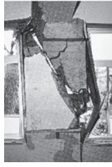
Figure 1. RC column whose axial load might decrease, 1995 Kobe earthquake (AIJ, 1997)
