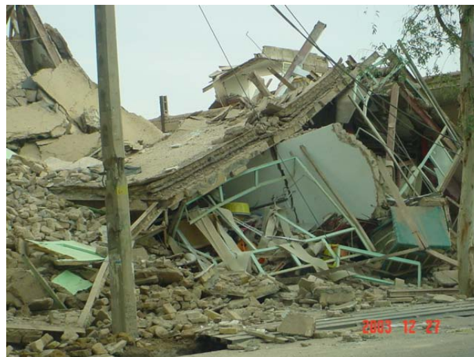
Figure-1: Bam after the disaster of Bam earthquake of 26/12/2003, Mw6.5 (photo by M. Zare, 27 Dec 2003).
