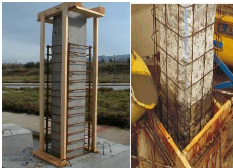
Figure 01: reinforced concrete jacketing of columns ( BRGM, 2006)
