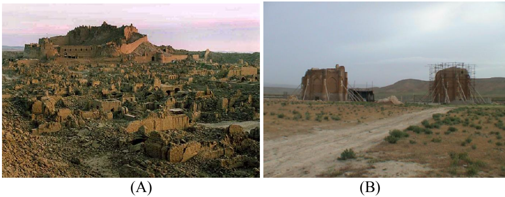
Figure 3. Damages caused by the earthquake to: (A) Bam Citadel in Bam Earthquake of 2002; (B) Kharaghan Twin Tower in Avaj Earthquake of 2002
