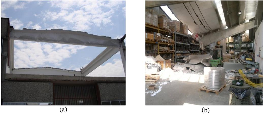
Figure 1. (a) Roof elements collapse due to the loss of support from main beam. (b) Loss of support of beam from column.
