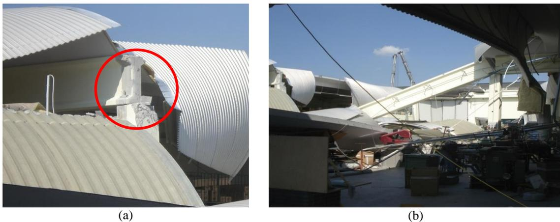
Figure 2. (a) Dowel beam-to-column connection failure and (b) consequent loss of support of the beam from column.
