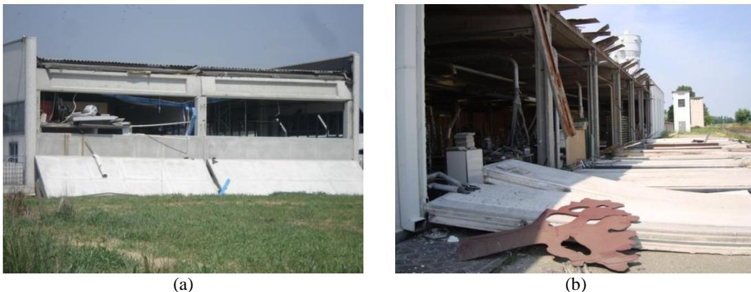
Figure 4. (a) Collapse of horizontal precast panels; (b) collapse of vertical precast panels.
