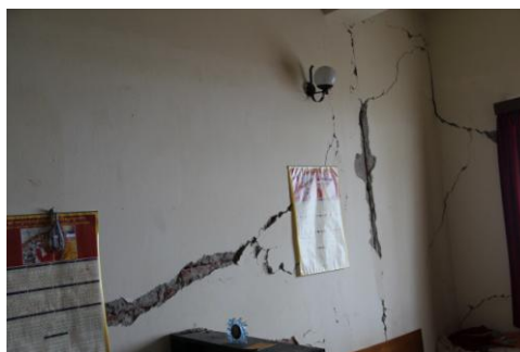
Figure 5. Diagonal crack
