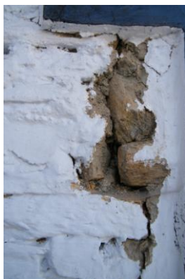
Figure 20. Crack on pier masonry Figure 21. Cracking of plaster
