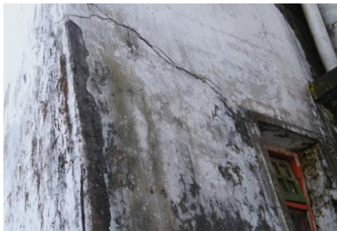
Figure 4. Corner crack
