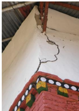
Figure 11. Flexible diaphragm action
