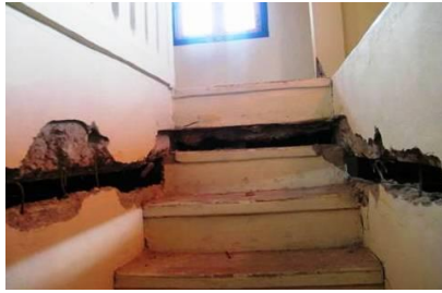
Figure 8. Disconnection of stair with floor Figure 9. Separation of unconnected wooden staircase
