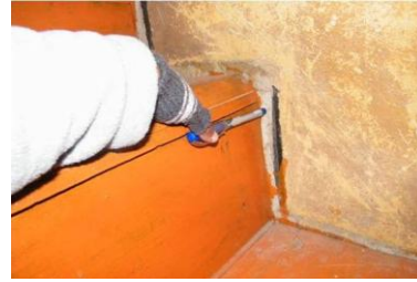
Figure 8. Disconnection of stair with floor Figure 9. Separation of unconnected wooden staircase
