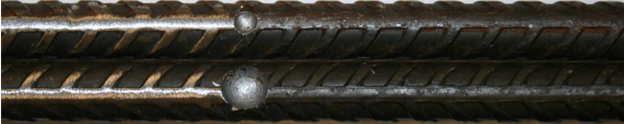
Figure 6: The sizes of pits on the surface of 10mm deformed bars
