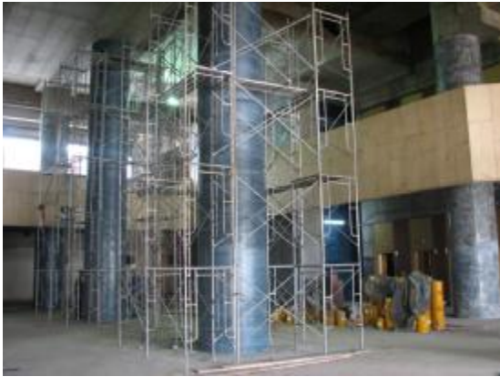
Figure 7. Strengthening of columns in the lobby floor by FRP
