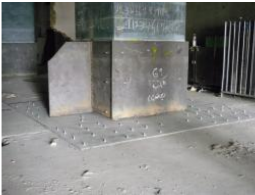
Figure 9. Strengthening of columns by steel plates
