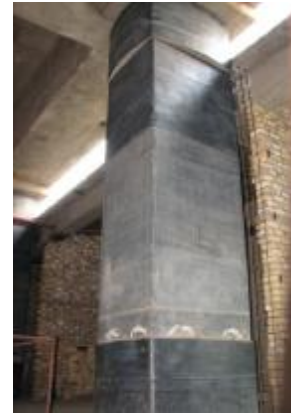
Figure 8. Strengthening of rectangular shape columns by FRP
