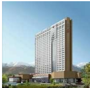
Figure 11. Azadi Hotel building after seismic retrofitting and architectural renovation
