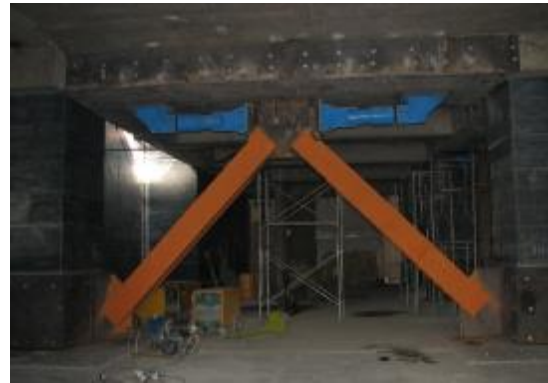
Figure 10. Executed bracing and damper
