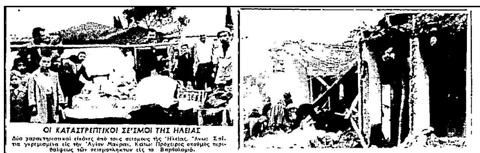
Figure 5: Two characteristic photos from the earthquake of December 23, 1954 earthquake. (Left) Collapsed buildings in Agia Maura. (Right) A collapsed medical centre in Vartholomio (ELEFThERIA newspaper)
