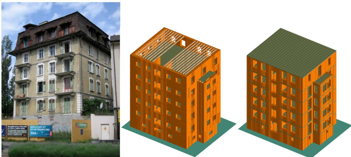
Figure 1. Study-building, numerical models before and after the retrofit work
