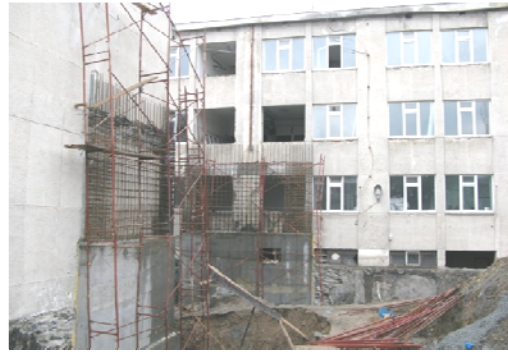
Figure 5. Construction of exterior concrete walls for a school retrofit
