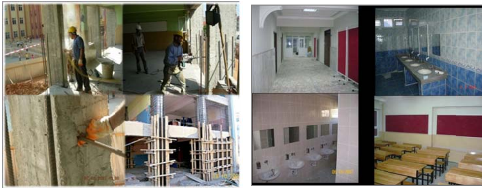
Figure 1. Retrofitting Works--Column Jacketing and Shear Wall and Implemented Renovation Works
