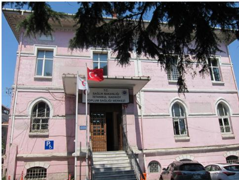
Figure 1. Front view of the building
