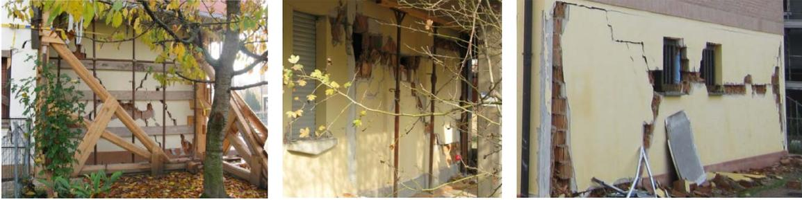
Figure 1. Examples of combined in-plane and out-of-plane masonry infill damage (Emilia, Italy - 2012)
