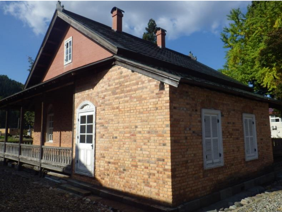
Figure 4. Masonry building (Ani Ijinkan, Akita, Japan)
