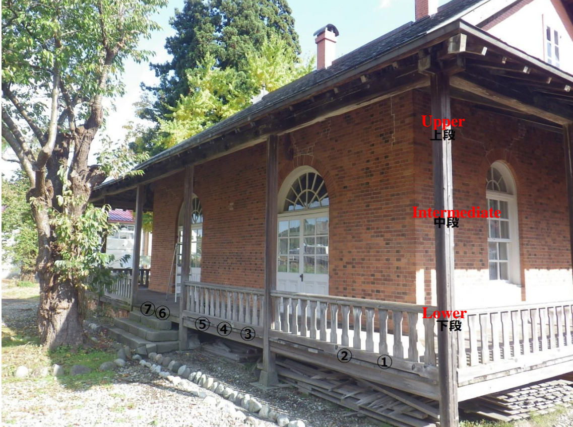
Figure 5. Determination of point of measurement for Schmidt hammer test
